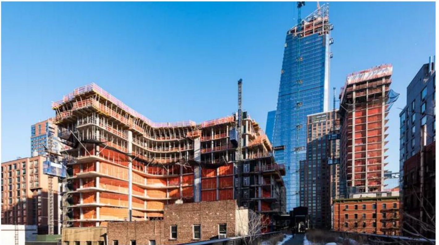
The Zaha Hadid-designed, under construction High Line condo building.
